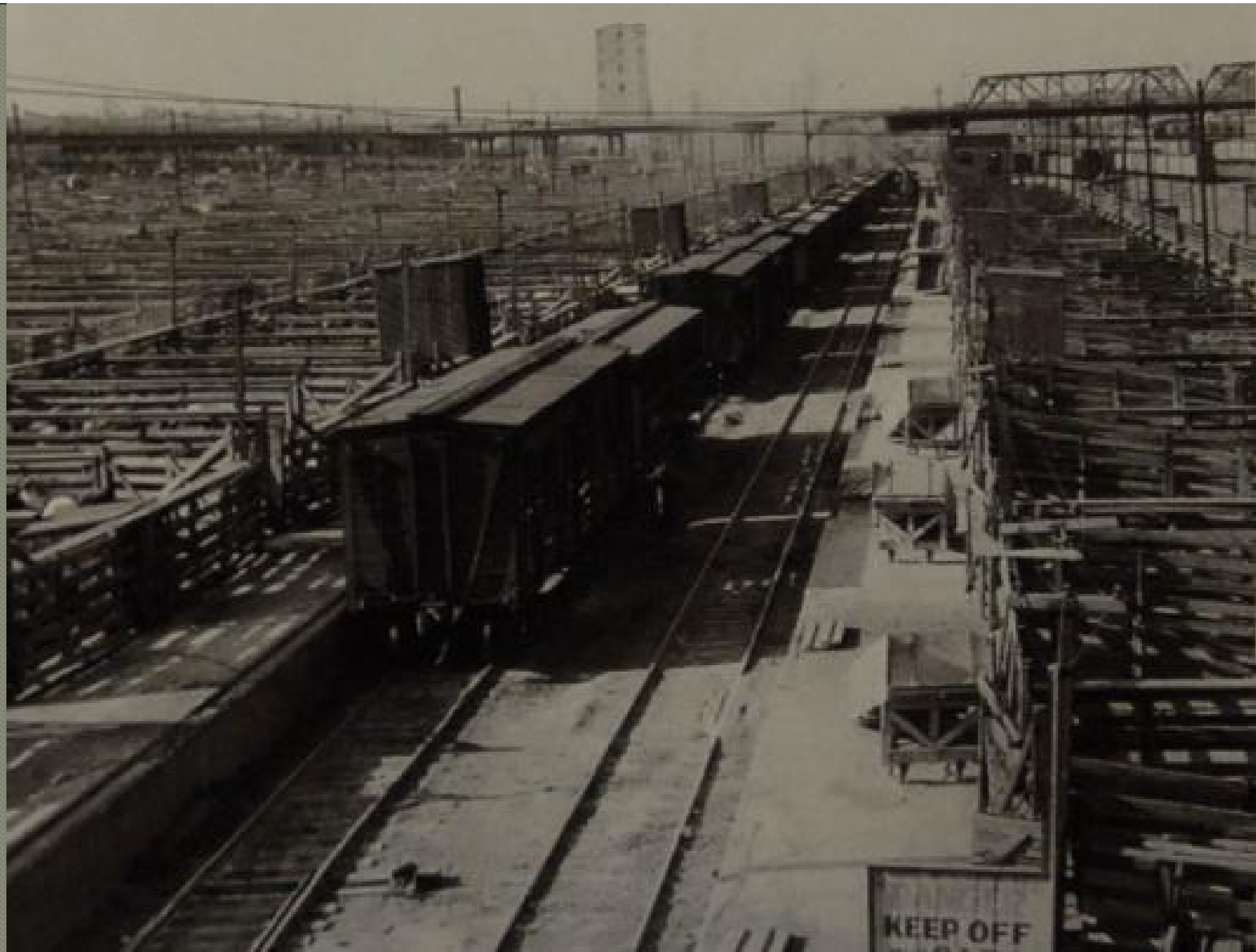
Car level loading platforms with movable chutes for upper decks, Omaha Union Stockyards (1941)
